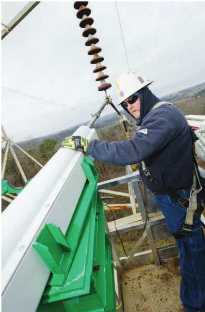
DSR installation on a TVA 161-kV transmission line.
