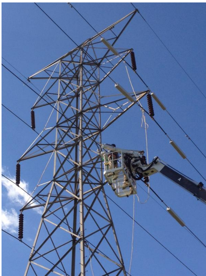
Picture 2: DSR Installation on High Voltage Overhead Lines (1)
