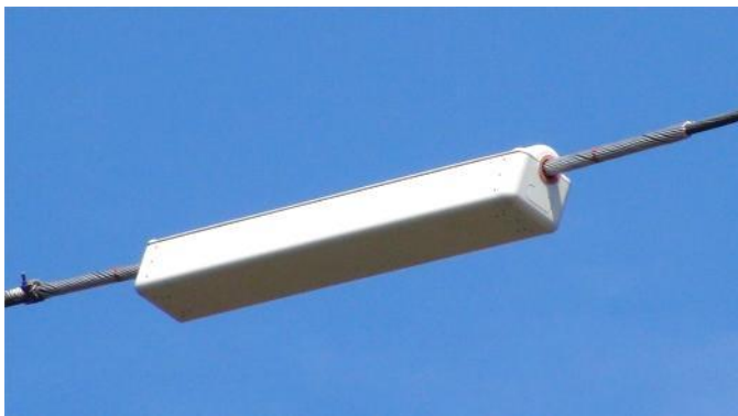
Picture 1: “Power flow controller“ – Distributed Series Reactor (DSR)
