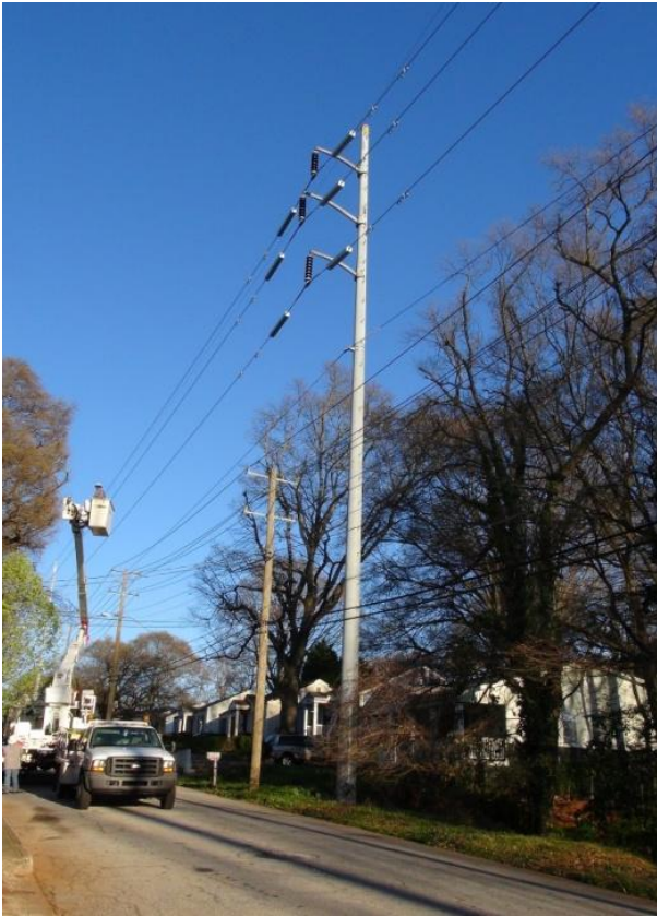
Picture 3: DSR Installation on High Voltage Overhead Lines (2)
